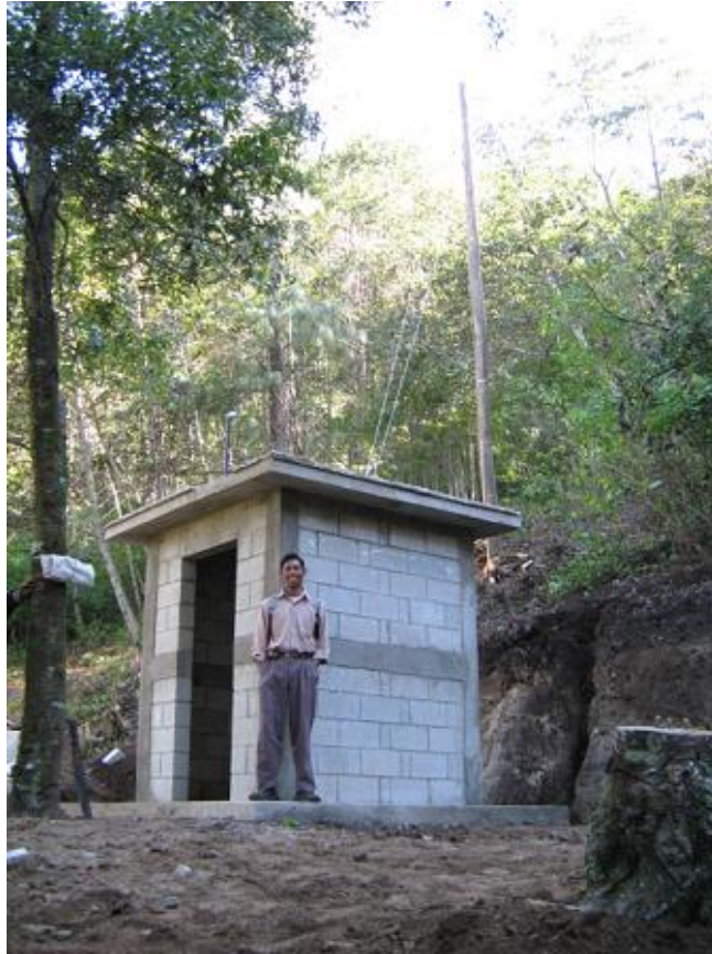
Alberto and the El Adelanto pump control cabin
