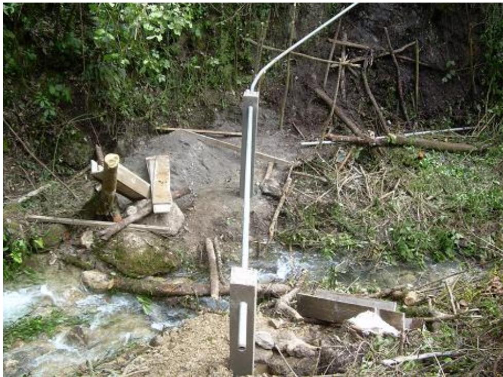
Kalampatzom conduction line stream crossing.
