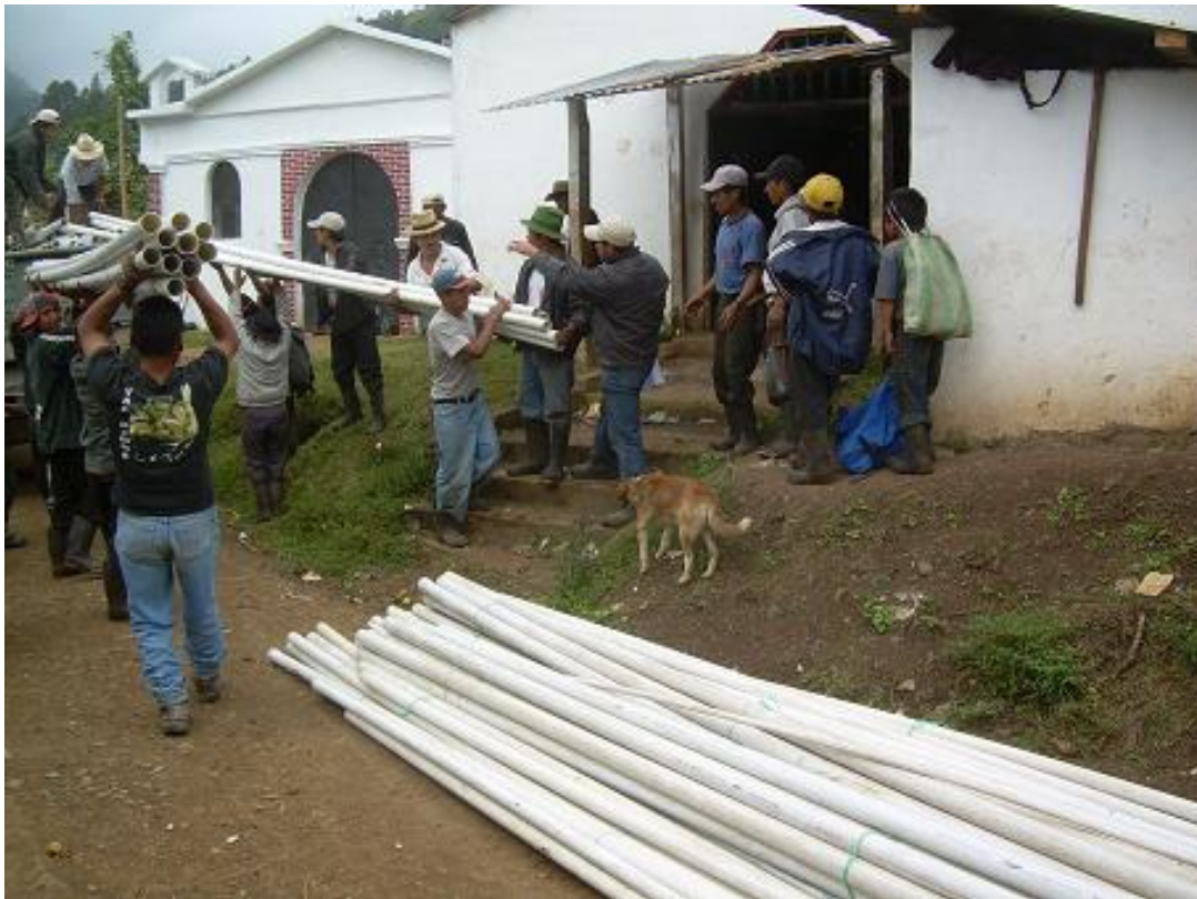
Unloading tubing for Kalampatzom pipe line
